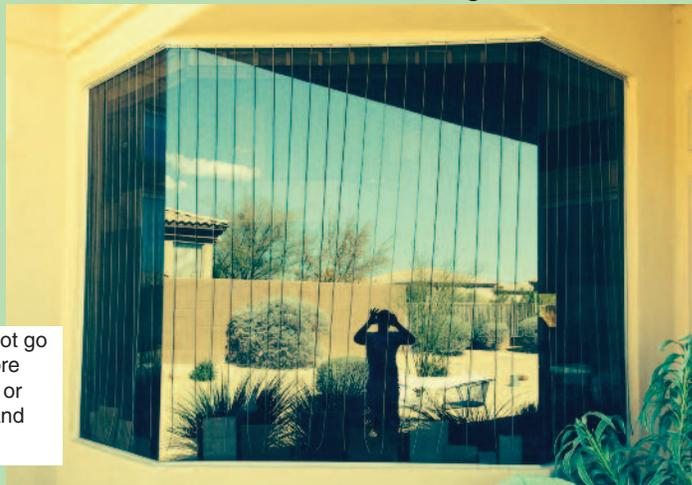
Option 1: Make the BirdSavers so the cords do not go all the way to the bottom of the glass. It looks more aesthetically pleasing when you can see an inch or two of space between the bottoms of the cords and the bottom of the glass.
